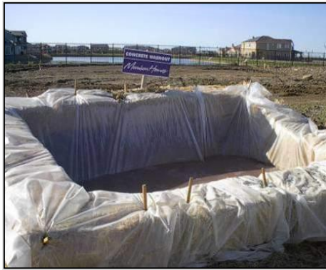
Plate 3-1 Typical concrete chute wash out areas
